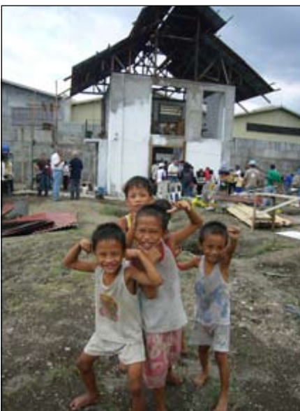
The new Material Recovery Facility taking shape.
